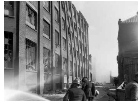
A view of Caley's chocolate factory looking towards the Chantry and the rear of the Assembly House, as firemen continue to work to damp down the fires.
