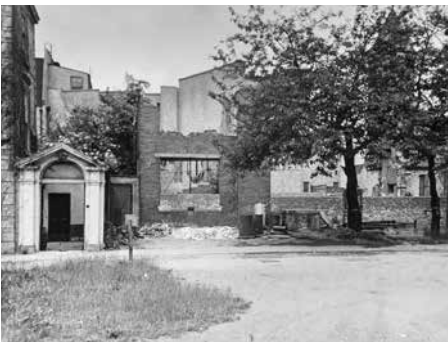
Blitz damage to the buildings adjoining the west wing.
