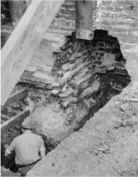
Above left: Working on the footings, 1949.
