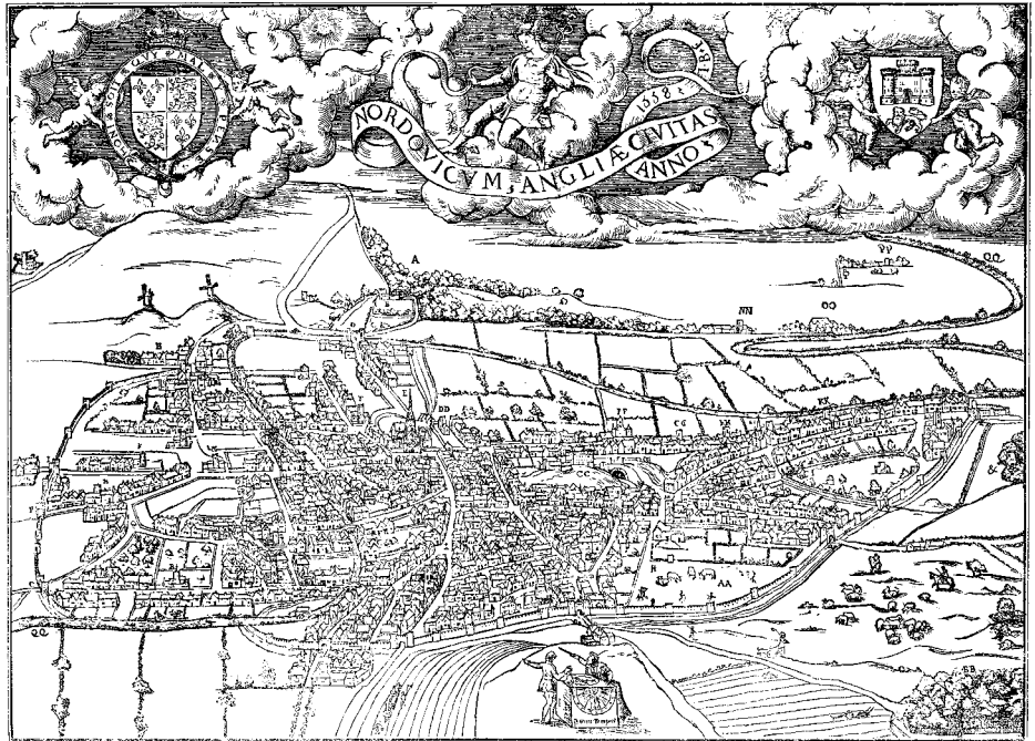
Cunningham 1558. The crypt and site of the chapel and college can be clearly seen in the bottom left, just inside the walls between St Giles' Gate and St Stephen's Gate.
