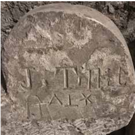
A piece of worked stone found in the crypt which appears to be a mason's mark and possibly an assembly mark. Did J. Tillit inscribe this on the hidden face of a piece pillar or vaulting or has it been repurposed as a gravestone?
